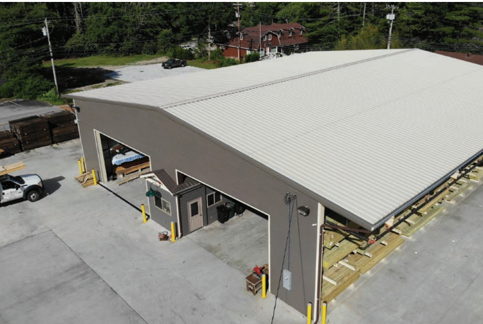
NORTH CAROLINA dealer created a drive-through structure to provide additional storage without additional overhead.
