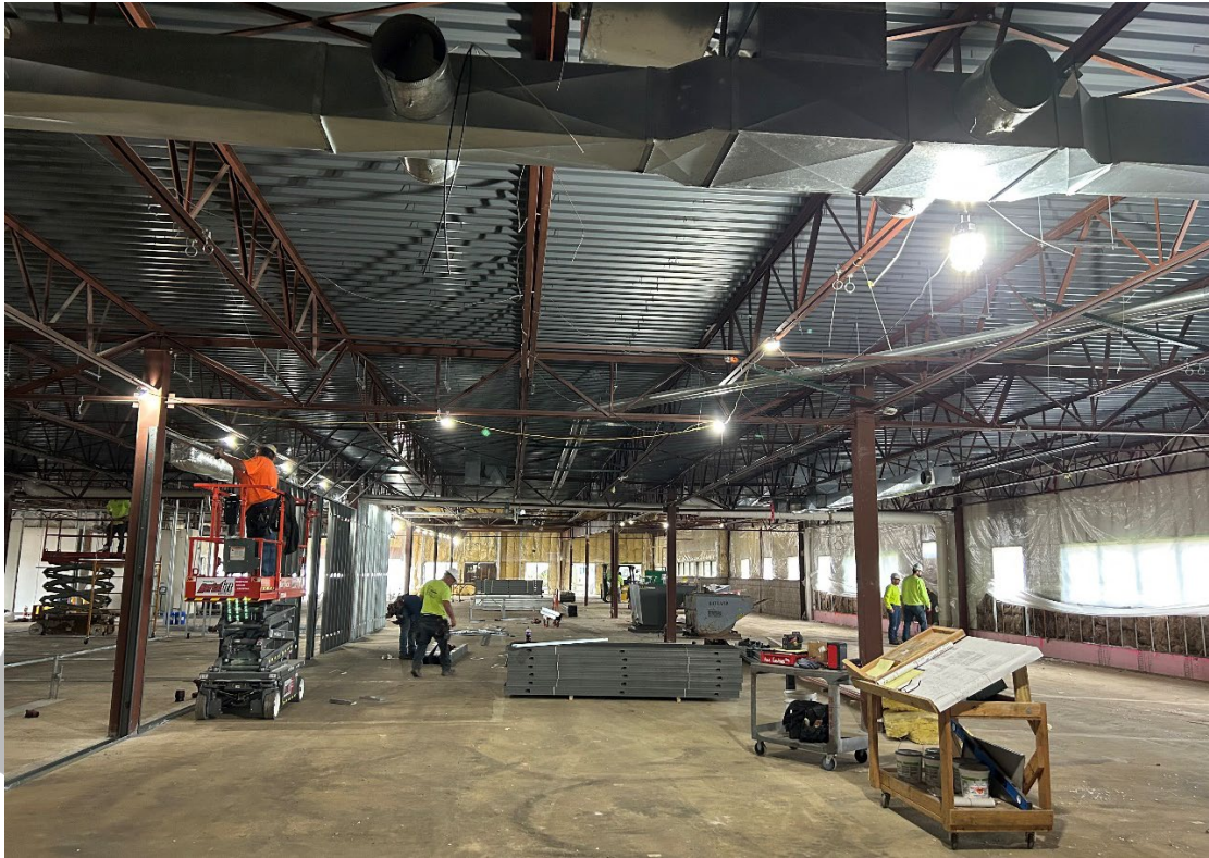
Interior construction of the new Steel King headquarters.
