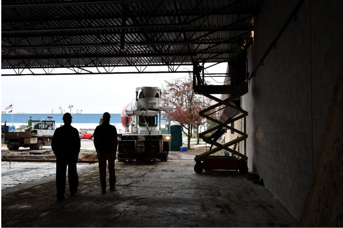
Construction underway of the new Steel King headquarters
